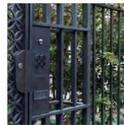
Railing (external) Location: To perimeter of gardens Product: N/A custom made metal railing with cast iron finials. Railing to match existing detail and railing on site by Palace Place Manufacturer: specialist blacksmith fabricator tbc Size: 2.1m high Colour: 'Invisible Green' (tbc)
